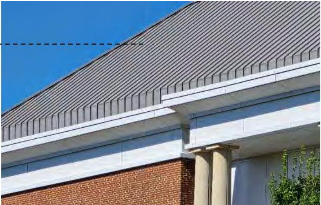
Zinc Panels at Data Hall and Roof Screen to Match Adjacent Buildings
