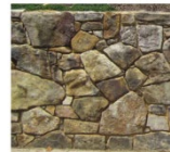
4 Trash Enclosure Wall With Stone Veneer
